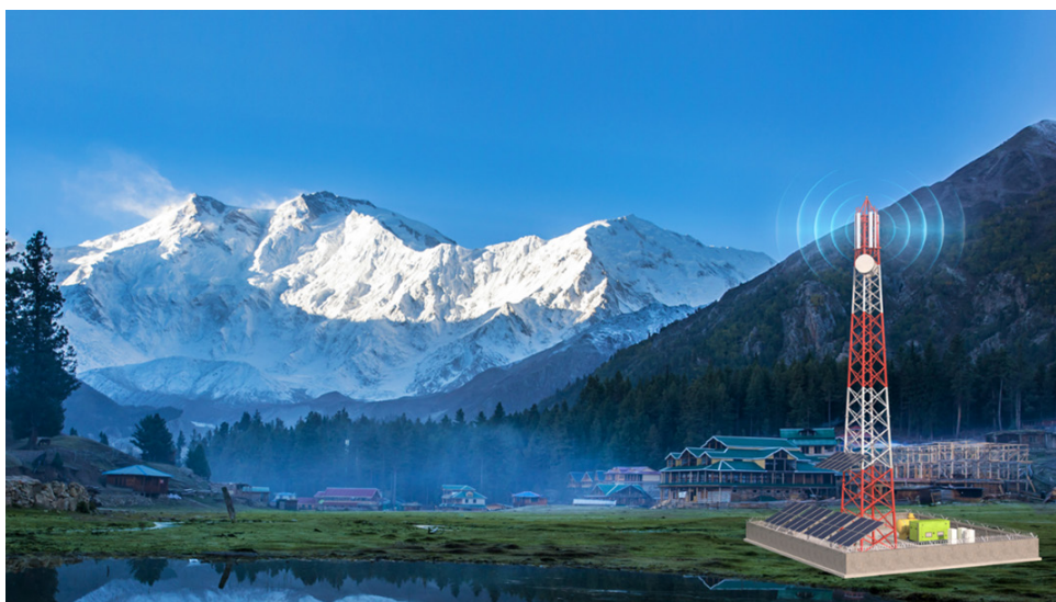
Upgrading sites with PV power in Pakistan
