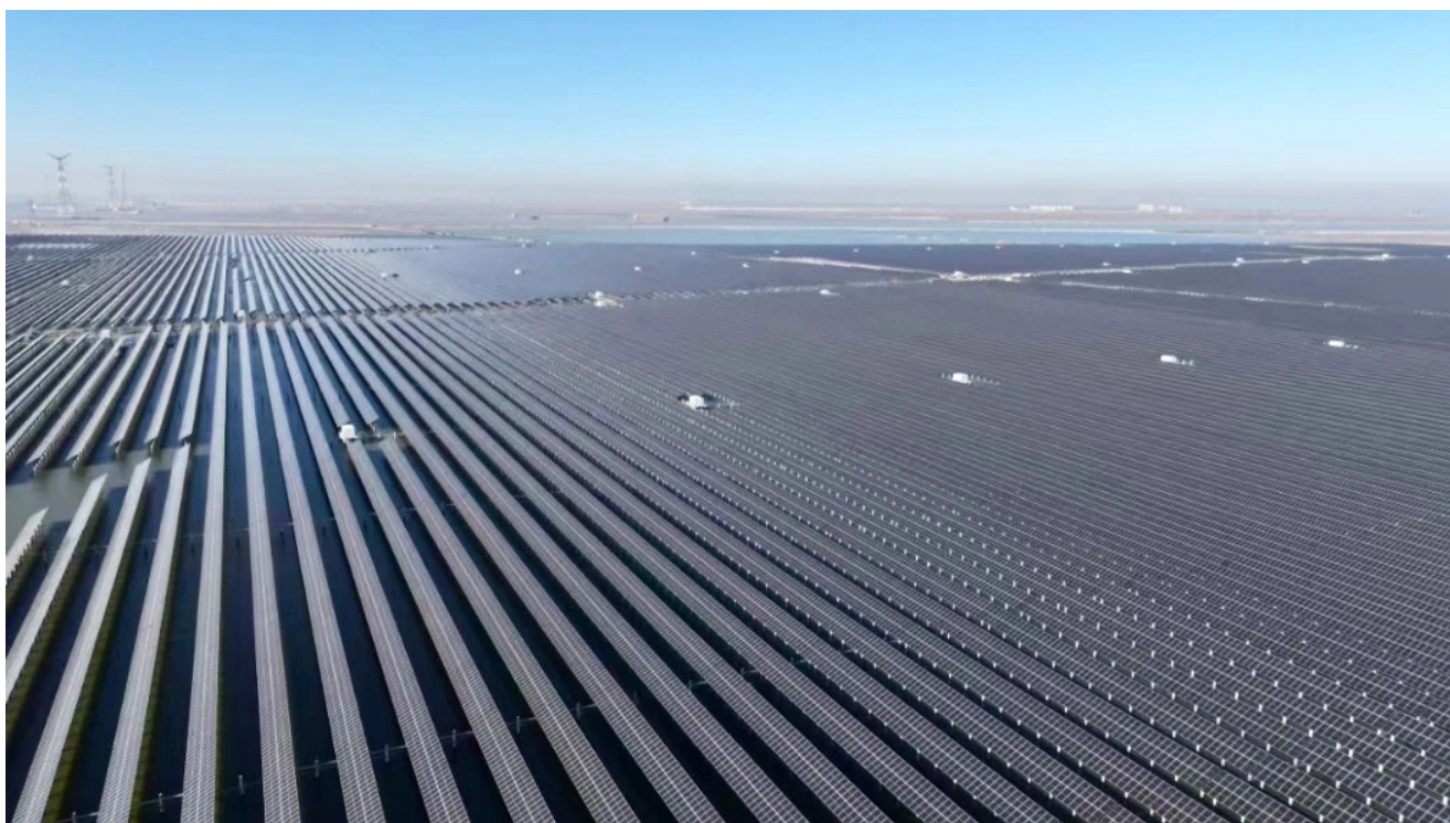
Huaneng Binzhou New Energy's project
